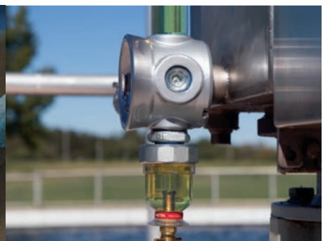
Clarifier - Wastewater Treatment Plant
