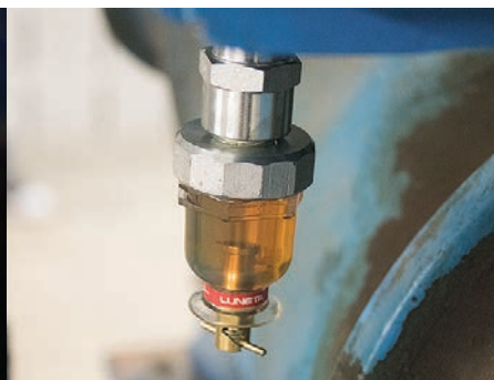
Large Blower - Wastewater Treatment Plant
